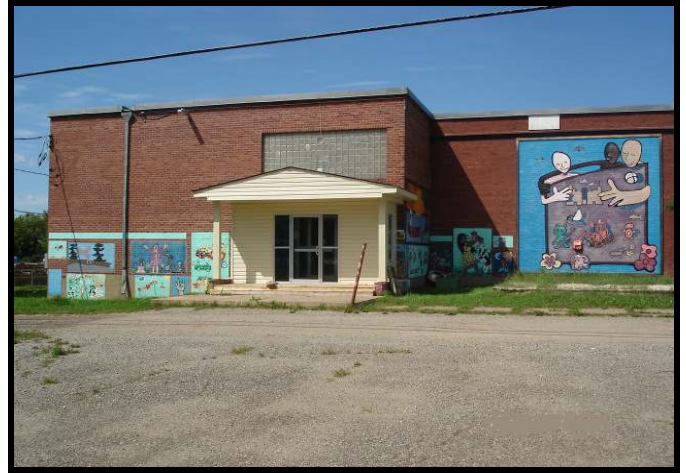
Double door entrance with security lock.
