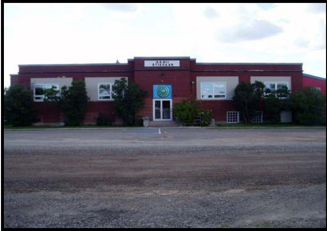
West side/back wall. Windows on both levels!
