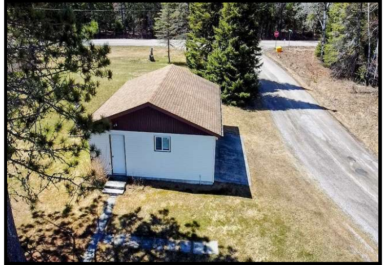
View of Detached Garage
