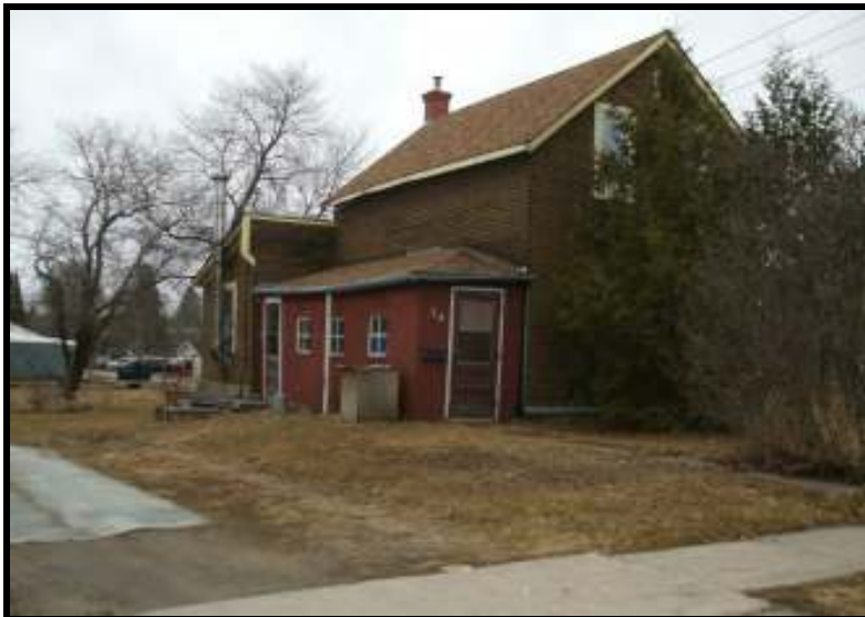
Home that needs to be removed, front view
